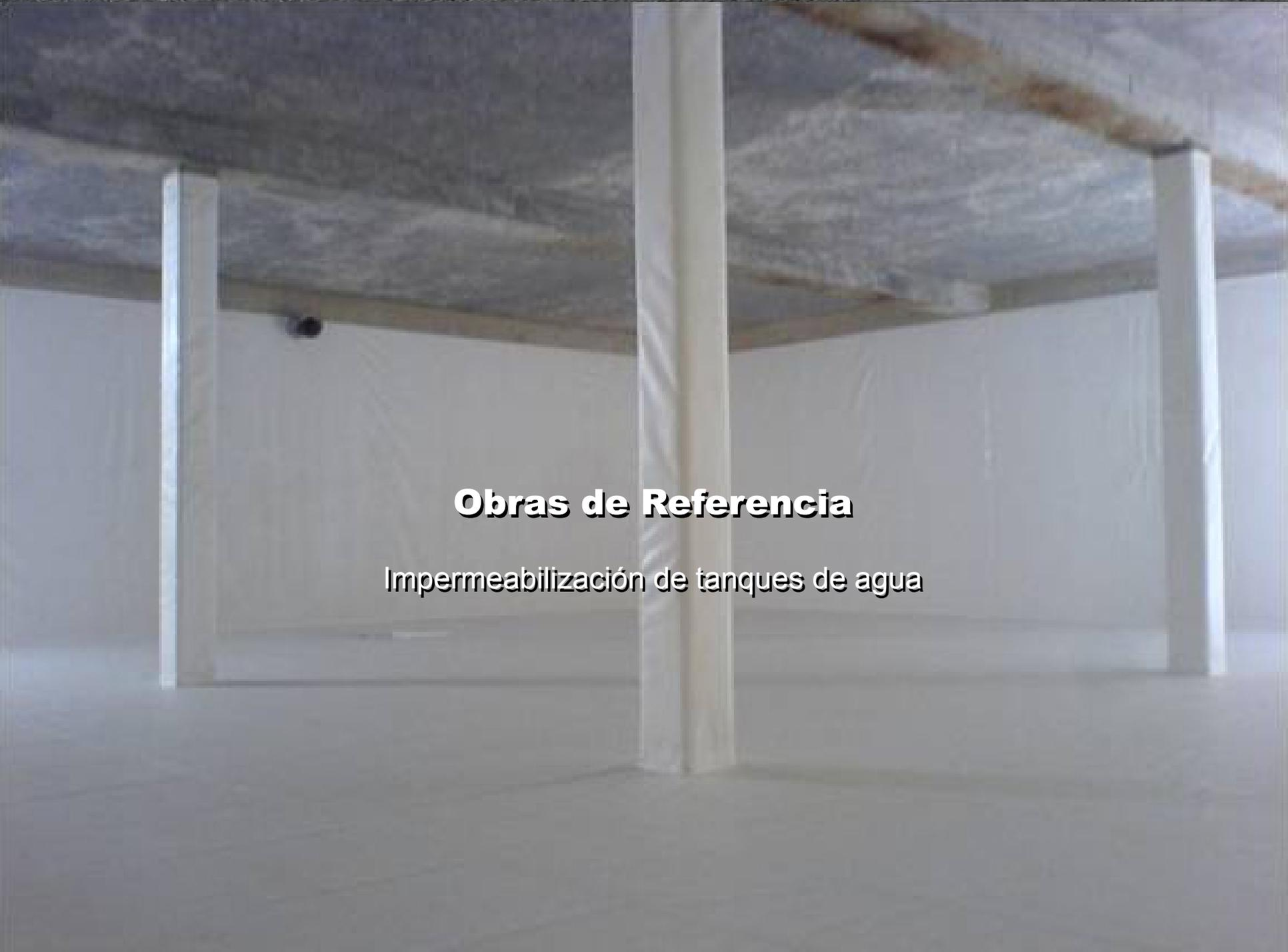
The image shows the interior of a large, empty concrete structure, likely a water tank, during a waterproofing project. The walls and ceiling are covered with a white, crinkled plastic membrane. Several vertical concrete pillars support the ceiling. The floor is a smooth, light-colored concrete. The lighting is somewhat dim, and the overall atmosphere is one of a construction site.
